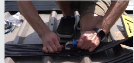
You may wish to shorten a coil because the roof is shorter in one section or to avoid a large obstacle (like a skylight). You need to perform these steps before the silicone adhesive is applied under the collector.
